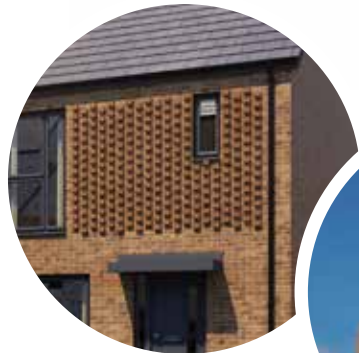
Brick Detailing & Slate Roofed
